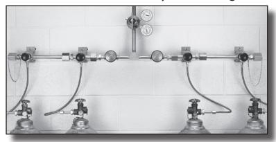
The 633 Series Duplex supports two banks of high pressure cylinders for applications where continuous gas supply is not required. A heavy-duty valve manually controls the bank priority, and line or station regulators should be installed at the point of use to ensure constant delivery pressure. Use of Acetylene requires flashback arrestor on pigtails. All fuel gases require flashback arrestors.
