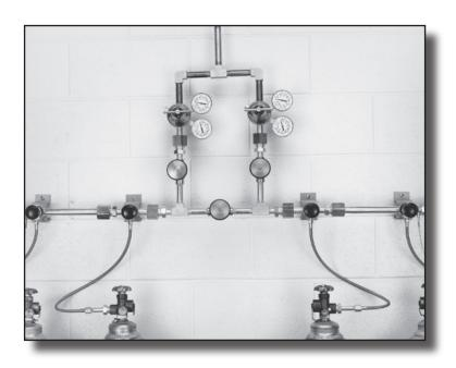
The 634 Series Switchover provides a continuous supply of gas through 2 extra heavy-duty 6700 Series regulators. Line or station regulators should be installed at the point of use to ensure constant delivery pressure. Use of Acetylene requires flashback arrestor on pigtails. All fuel gases require flashback arrestors.
